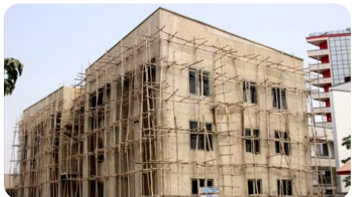
The Poly Clinic Building Under construction
